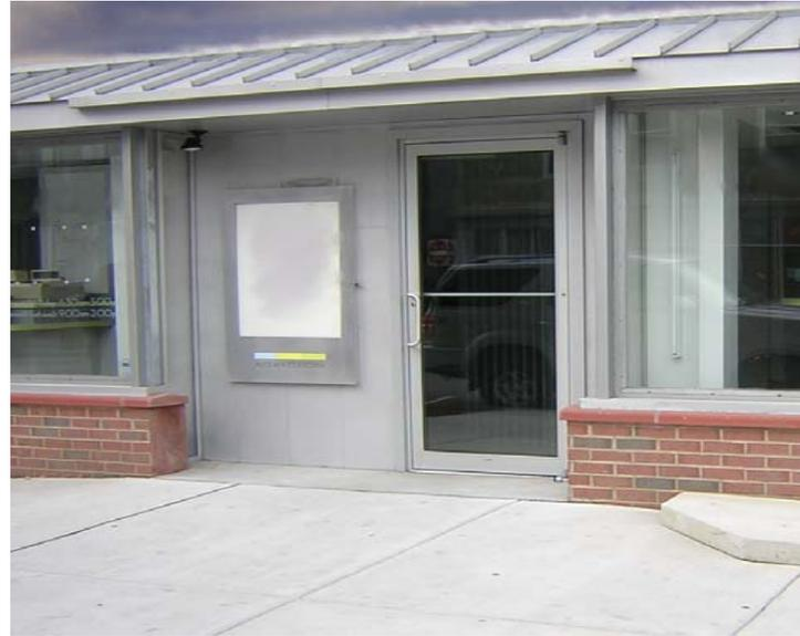
The photo on the left shows a two-inch high threshold. Although only a small rise, the threshold creates a significant barrier for a person using a wheelchair.
